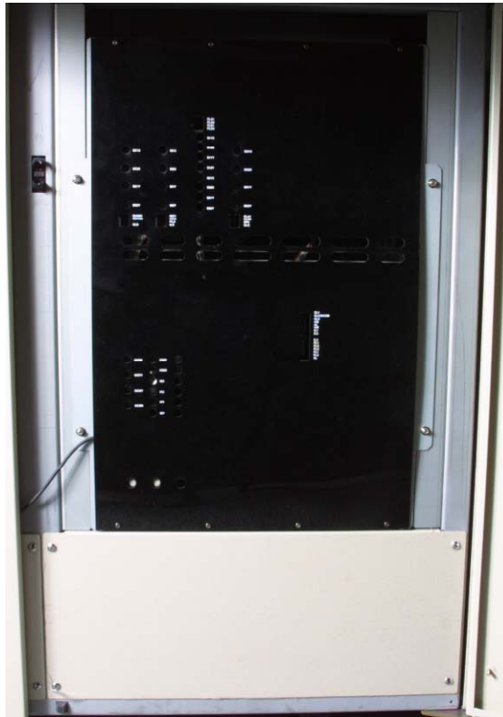
Fig. 4.6 Control panel R2
